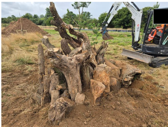
Image 22: Vertical log piles
